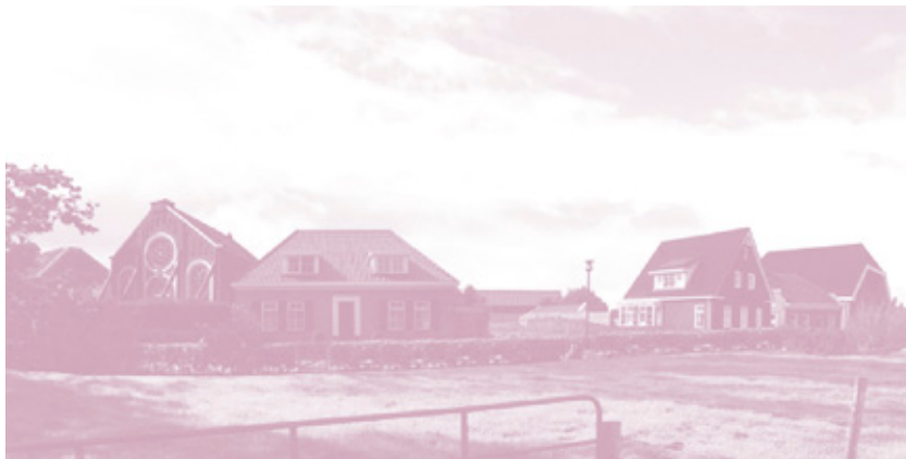
Figure 2. After the reinforcement measures and demolition
